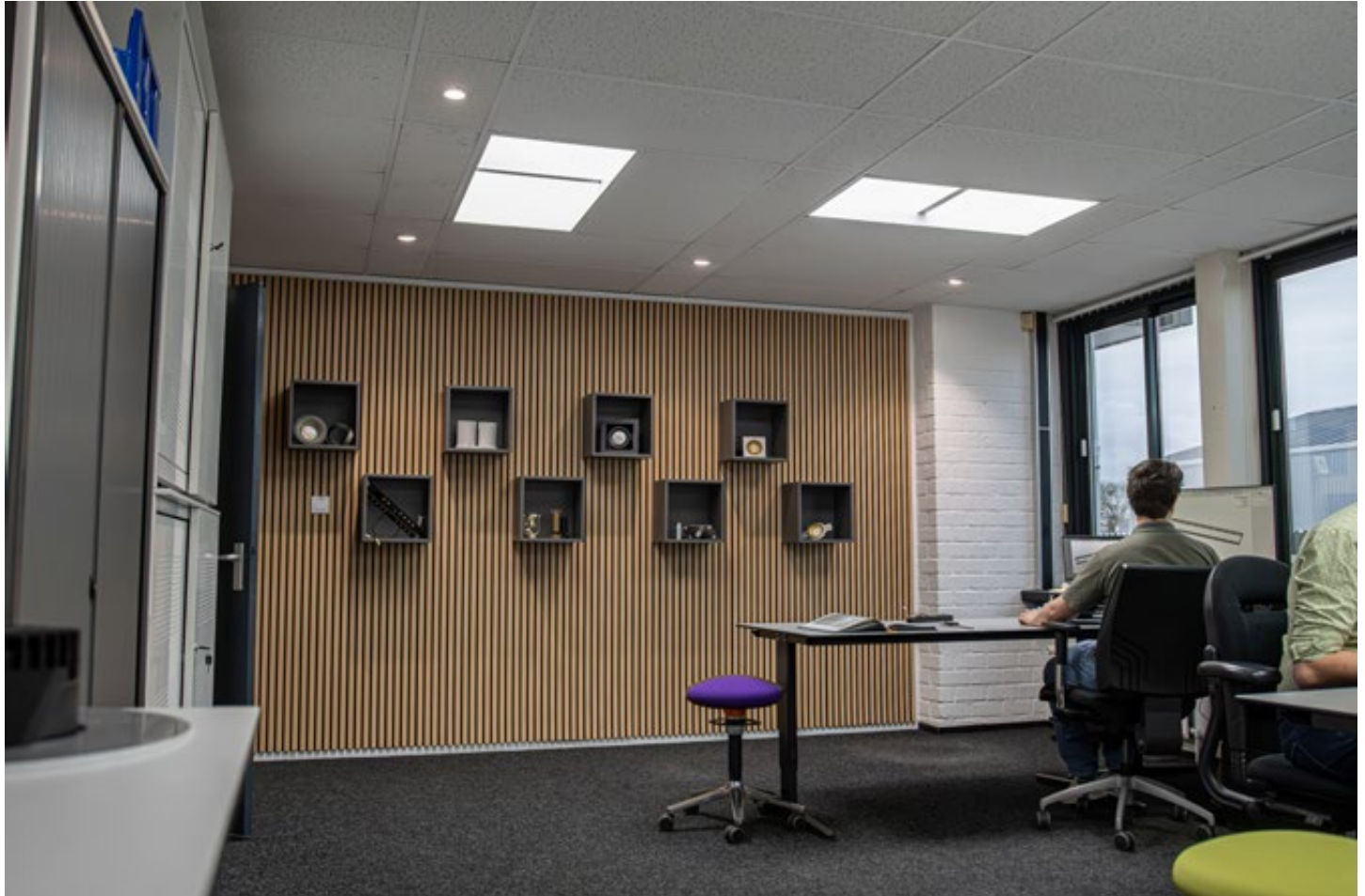
The lighting plan consists of two lighting groups. The panels provide a high mDER value for the eyes, while the downlights create comfort for the employee. Both groups operate independently to create a dynamic atmosphere.
